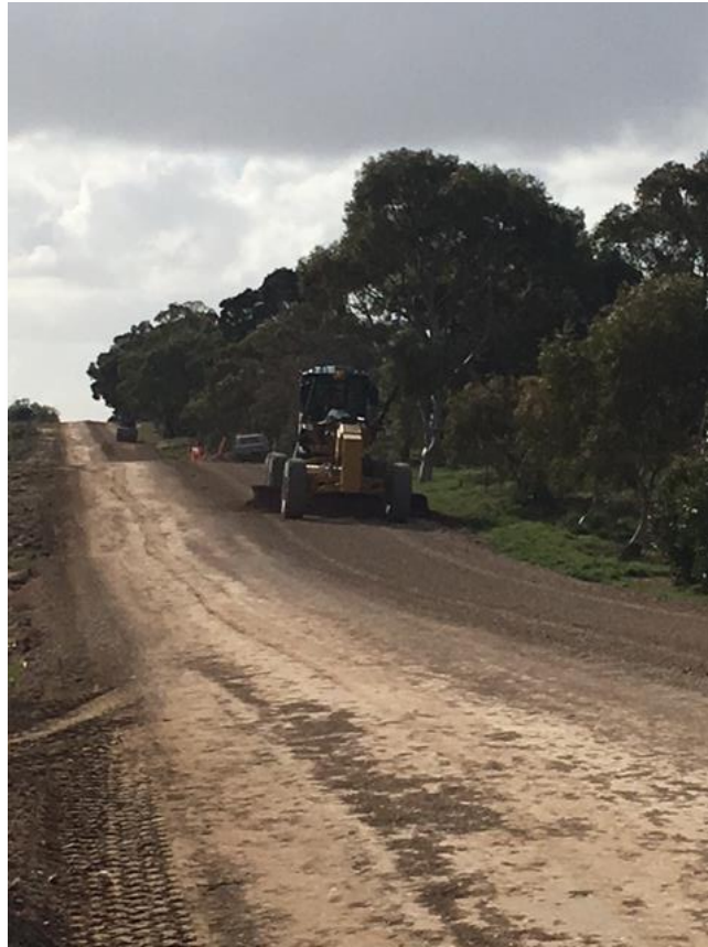
Pictured: Resheeting of Pangarinda Road
