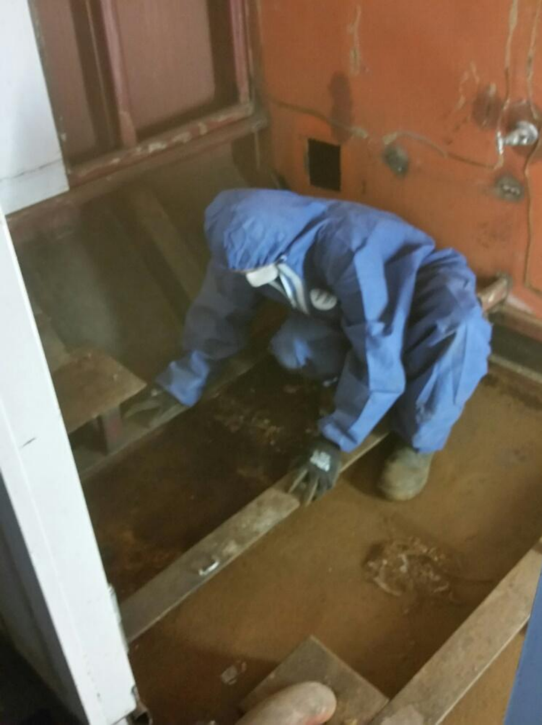
Asbestos worker in the hull of the Murray River Queen
