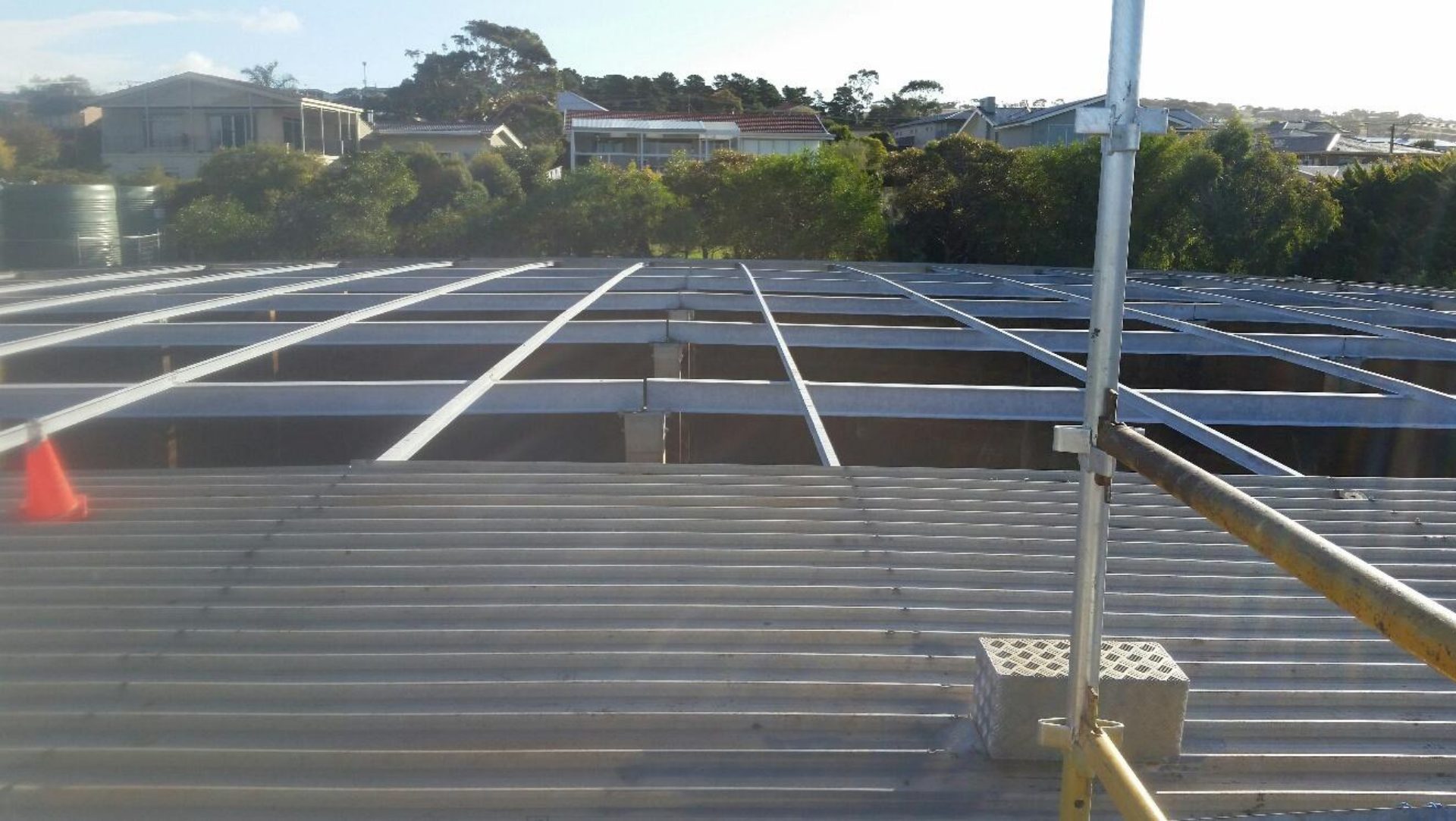
SA Water steel tank lid removal with asbestos mastic joins
