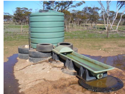
This trough fills in 60 seconds. Has 50mm float valve and pipe from tank
