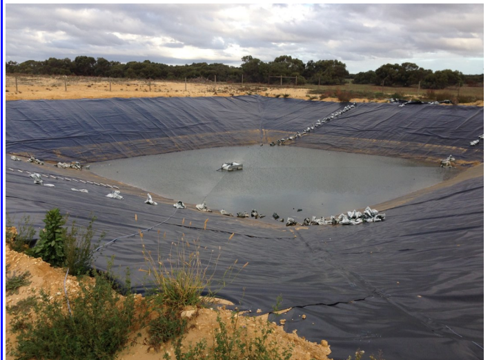
Completed dam with floating pump.
