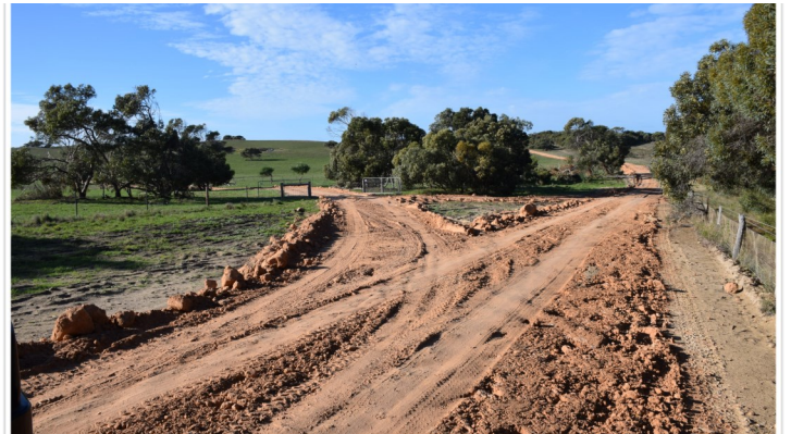
Excess rock was used around troughs and on roads The site must be rock free or liner damage may occur
