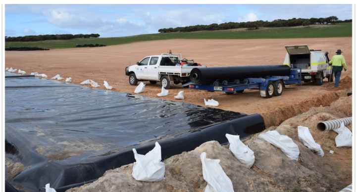
Poly liner initially weighed down with sandbags
