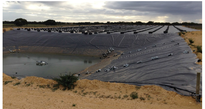
The liner needs to be weighed down to prevent lifting in the wind.
