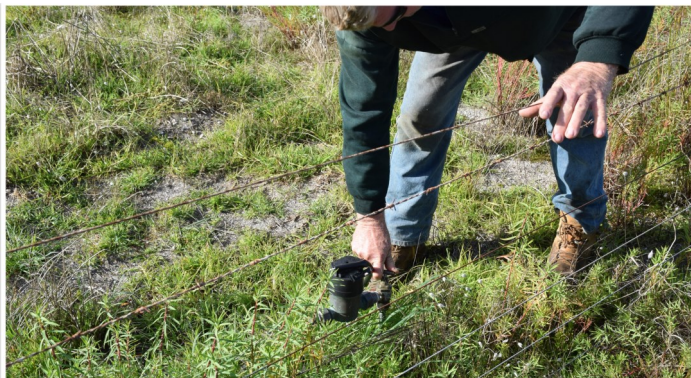
Mark turning off his SA Water meter.
