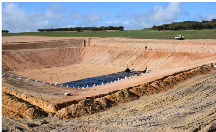
Commencing the instillation of the liner and the anchor trenches are clearly visible in the foreground.
