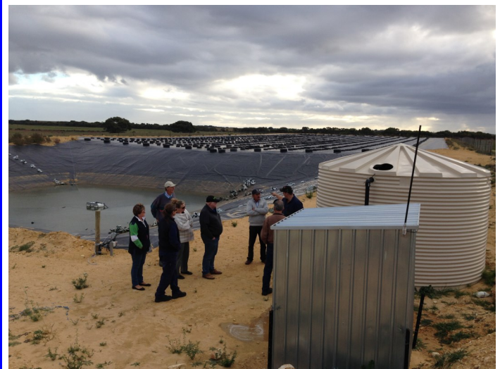
Pump shed and storage tank.
