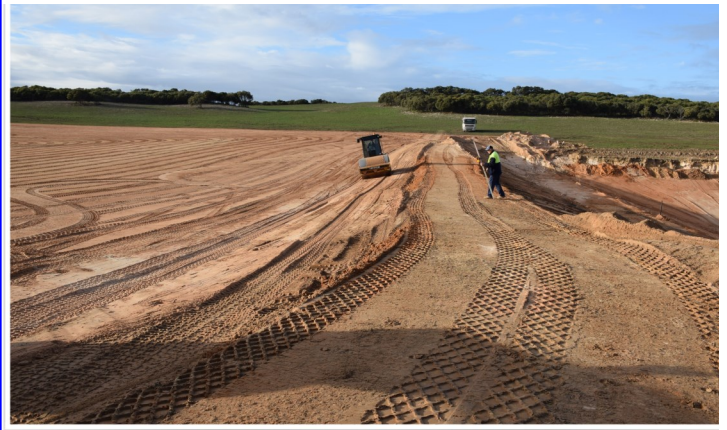
The whole site must be free of rocks and other debris otherwise liner damage may occur.
